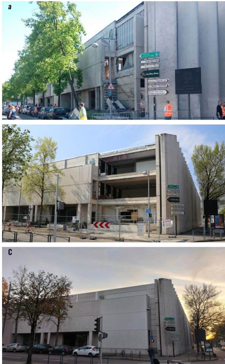
Figure 136 Photos of Nancy School of Architecture: a - view of the façade after the accident, b - view of the façade during the reconstruction, c - view of the façade after the reconstruction
