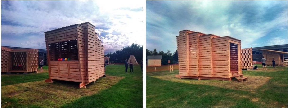
Figure 65 Timber Challenge 2018 project "Ramificarré" built by student team H
