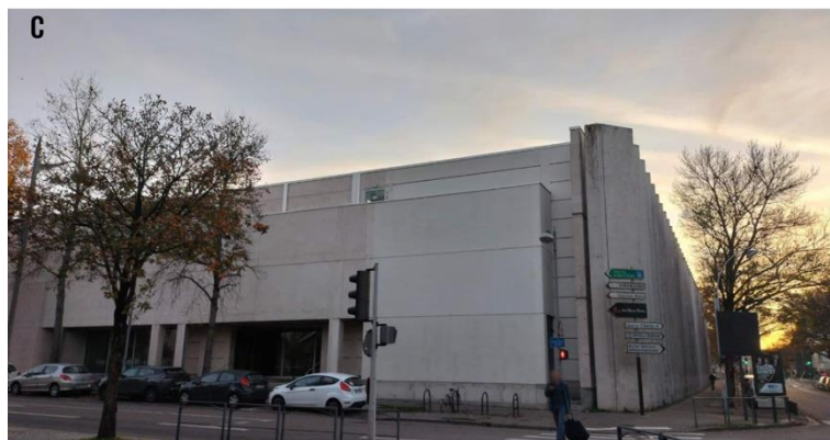
Figure 136 Photos of Nancy School of Architecture: a - view of the façade after the accident, b - view of the façade during the reconstruction, c - view of the façade after the reconstruction
