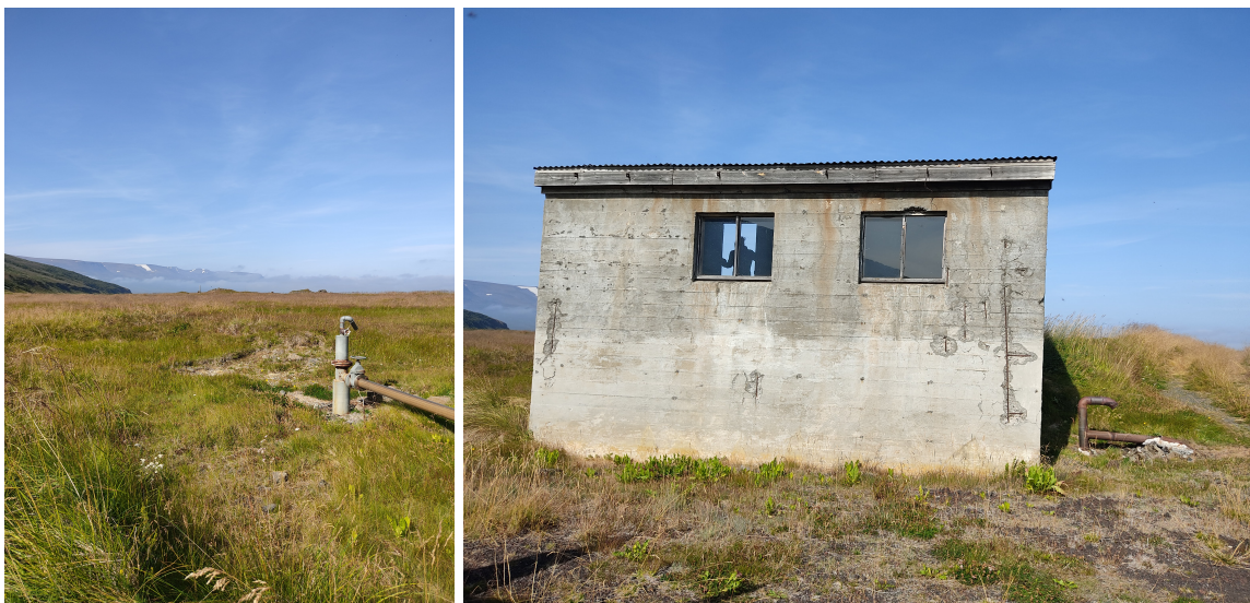
Figure 1.10: HA-01; well head on the left and main building, where SPARTAH was connected and stored, on the right.
