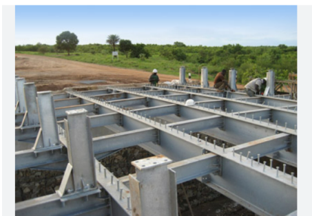
Figure 1.1 – Highway beam bridges construction.
