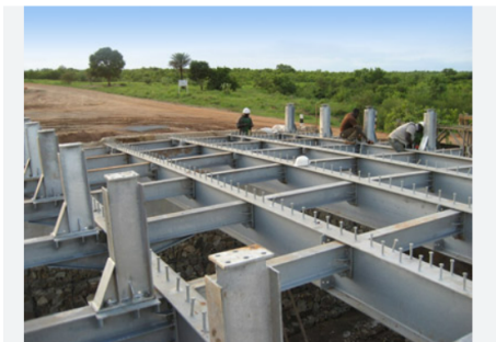
Figure 1.1 – Highway beam bridges construction.
